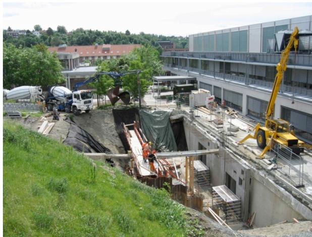
Digging of hole for 2000 hp (horsepower) back-up power generator
